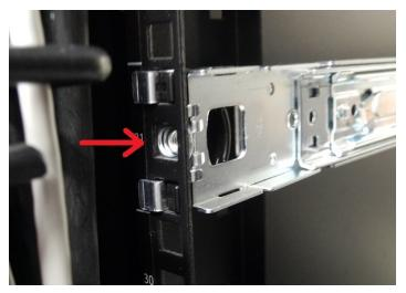
4. Fasten the transformer bracket to each sliding mount with two wide flat-headed screws.
