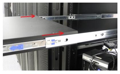
7. The HSM now moves smoothly and securely on the rails. Push the HSM all the way back and secure it to the transformer bracket with four rack screws.
